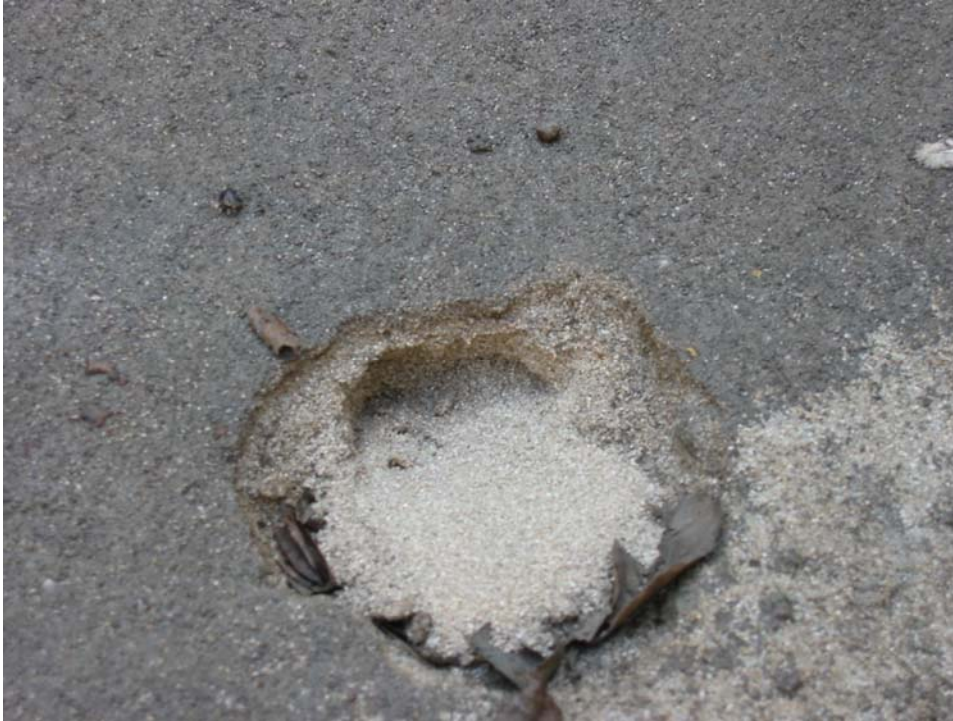
Figure 7 Formation of Clogging Crust on Filter Bed
