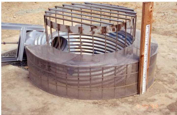
Figure 1 Example of Extended Detention Outlet Structure
