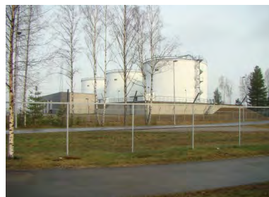
Figure 18 - OSL Fuel Tanks
