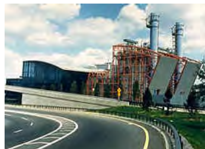
Figure 15 - Boilers at JFK
