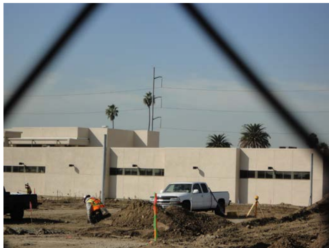
Jefferson Elementary School, October 2014 Construction of new section of the school
