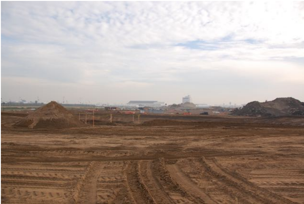
Figure 1.2.3-2: WAMA Construction Site
