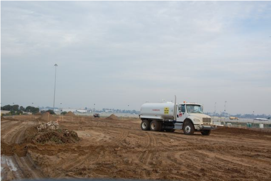
Figure 7-1: Dust Control Being Conducted on WAMA
