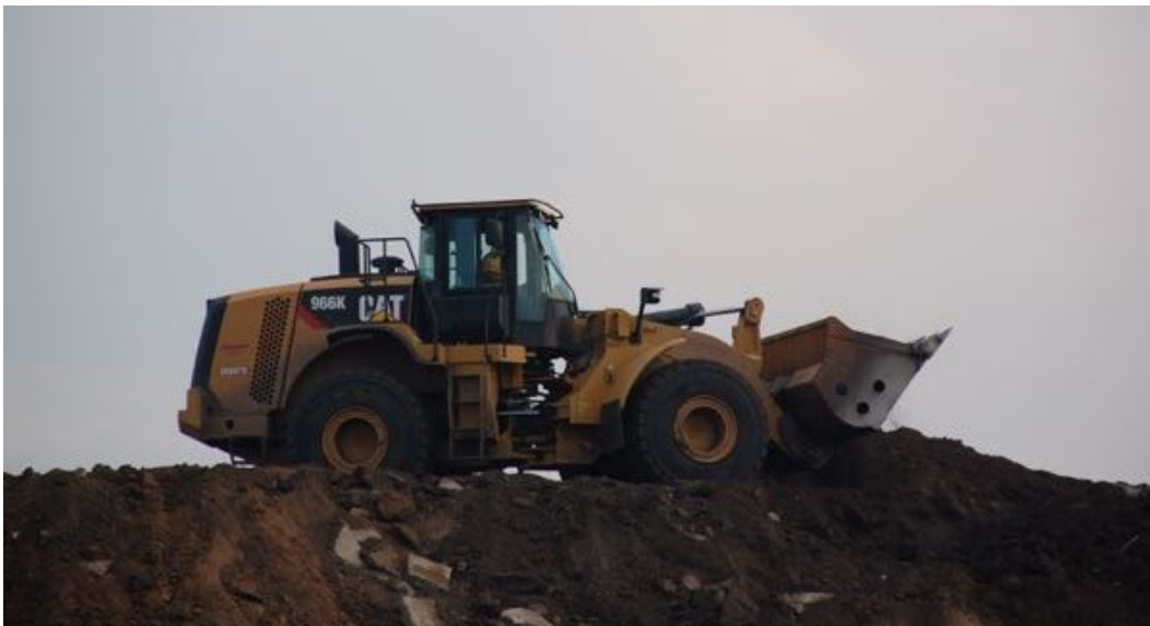
Figure 1.2.3-3: WAMA Construction Progress – Tier 4 Final Equipment in Use
