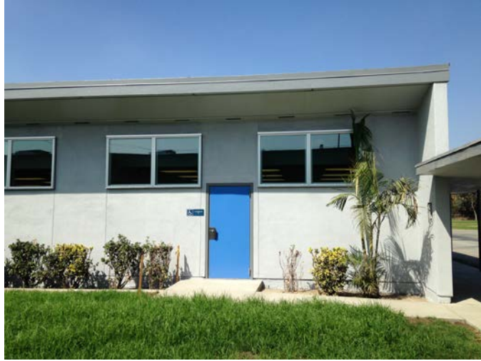
Felton Elementary School, September 2014 New double-paned windows and solid doors
