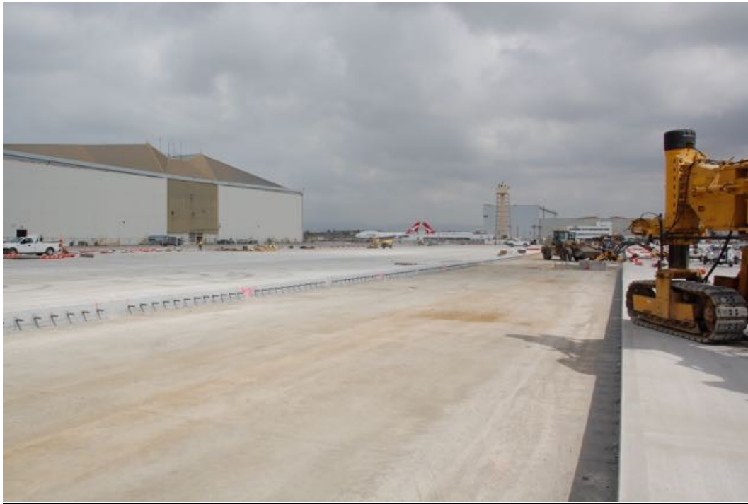
Figure 1.2.1-4: Taxiway T Phase 1 Construction in Progress – June 2014
