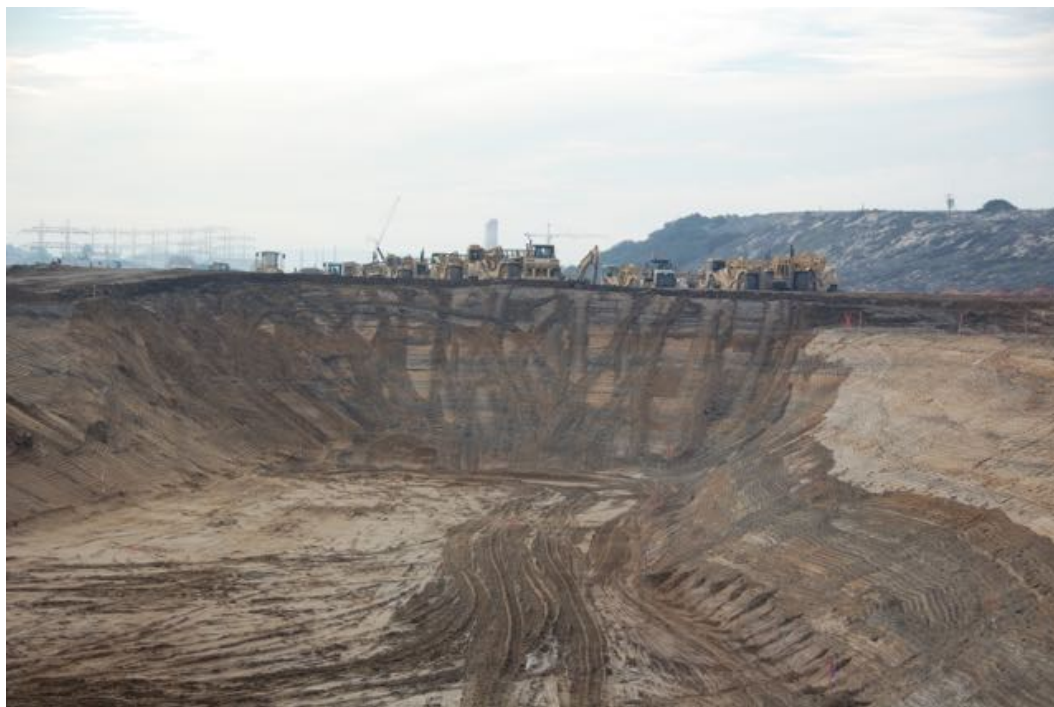
Figure 1.2.4-1: Qantas Hangar Construction Site
