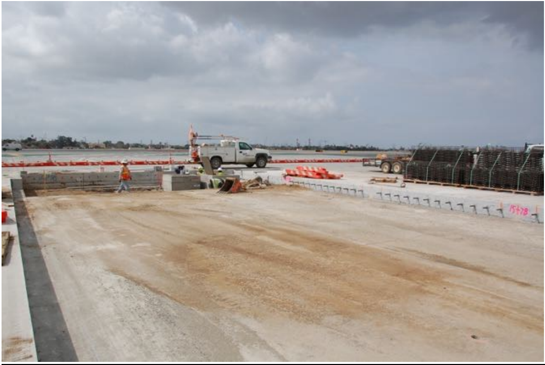
Figure 1.2.1-3: Taxiway T Phase 1 Construction in Progress – June 2014
