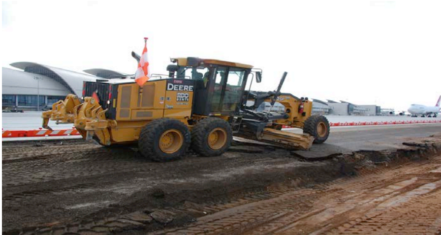
Tier 4i Grader Operating on Taxiway T
