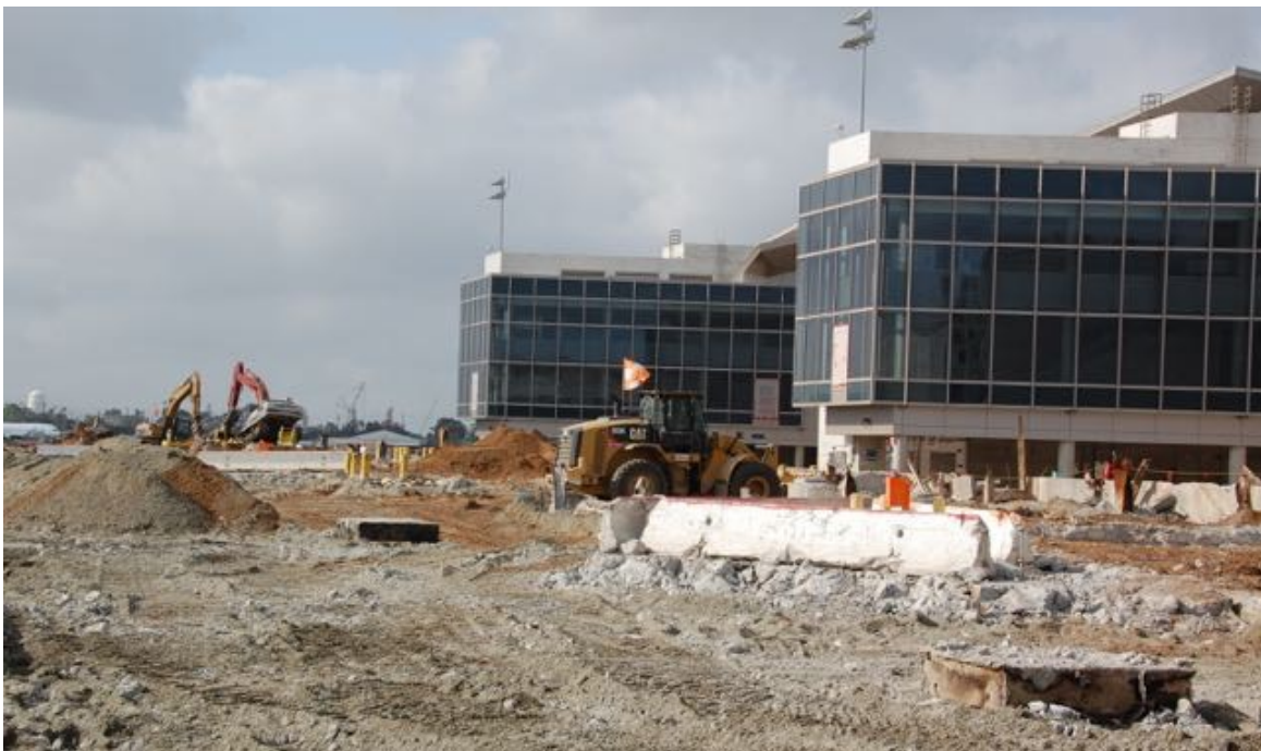
Figure 1.2.2-2: TBIT – East Apron Construction Progress – Tier 4i Equipment in Use
