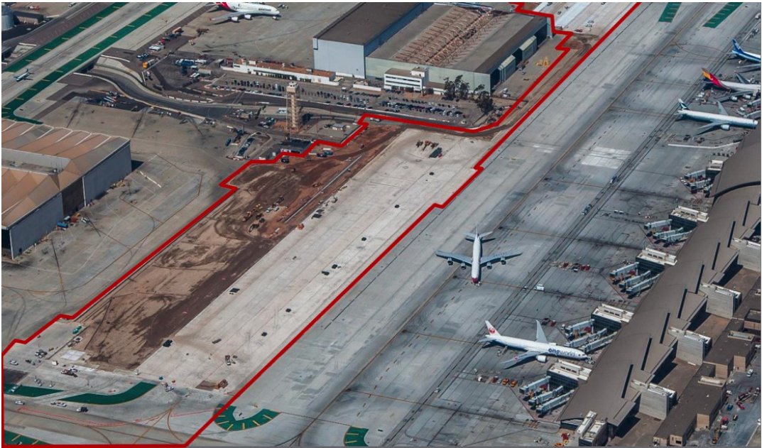
Figure 1.2.1-2: Taxiway T Phase 1 Construction
