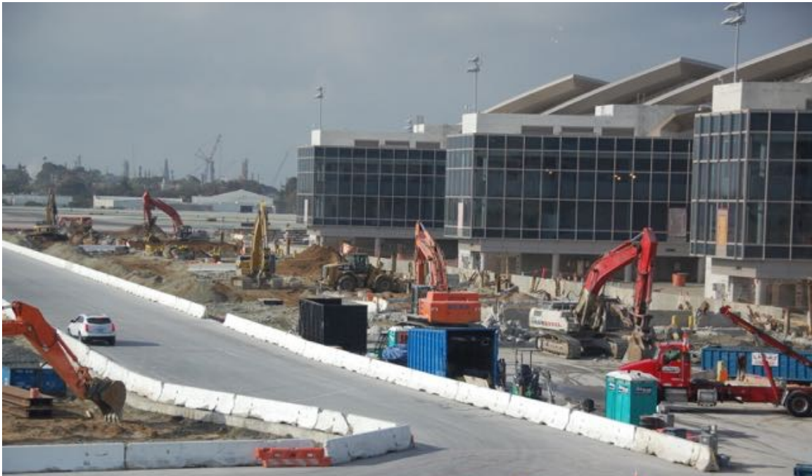
Figure 1.2.2-1: TBIT – East Apron Construction Progress
