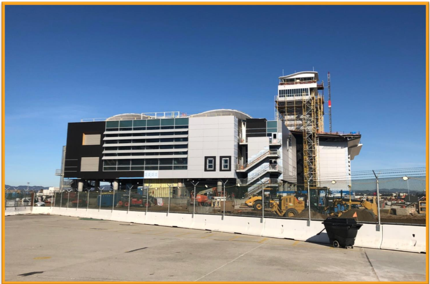
MSC North, featuring the MSC Ramp Control Tower, pictured from airside
