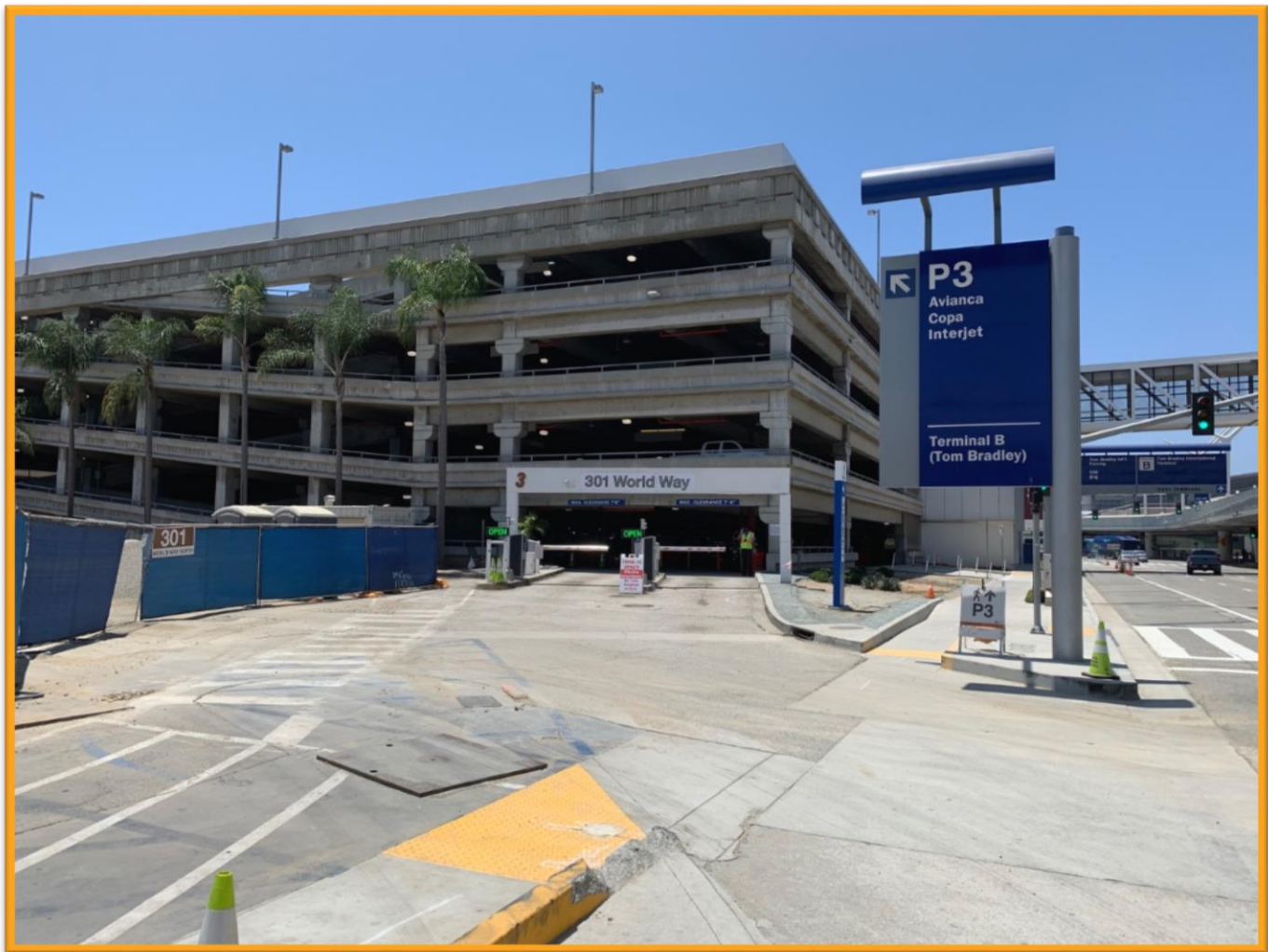
PS-3 entrance to be impacted by APM construction
