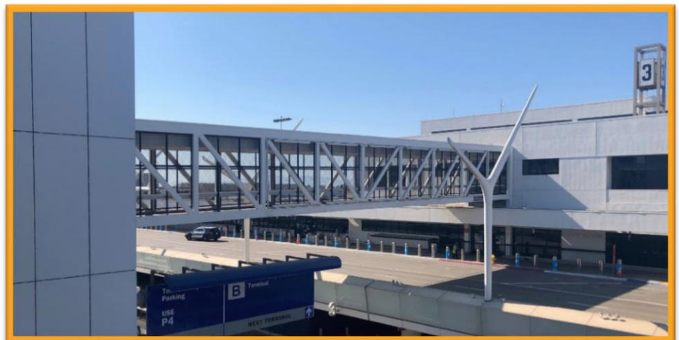
Pedestrian bridge to be demolished
