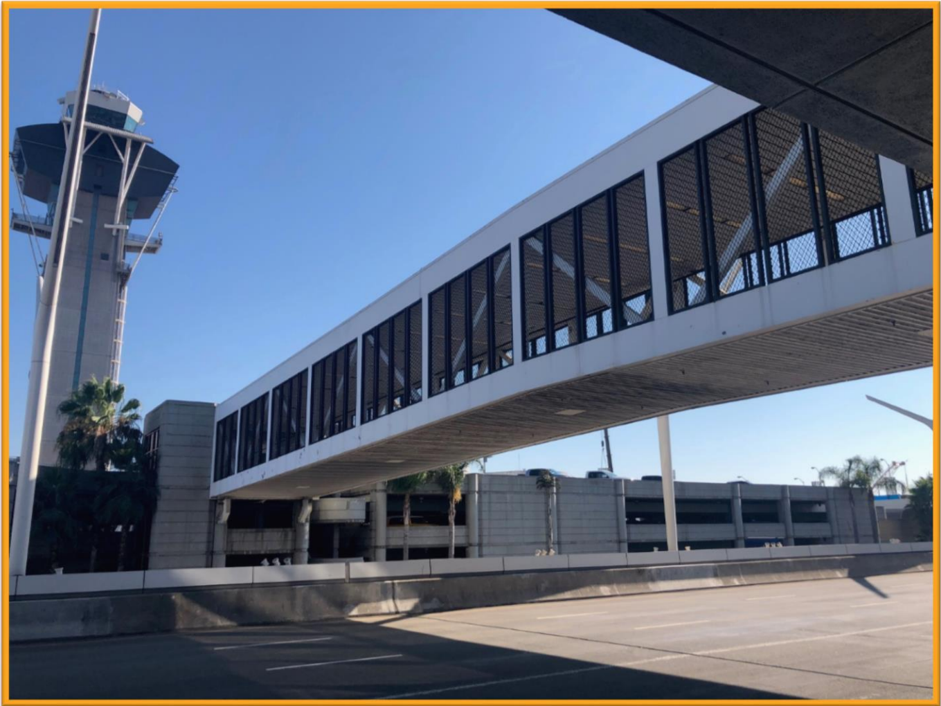
Pedestrian Bridge between Terminal 2 and Parking Structure 2A, pictured from the Departures Level roadway looking south
