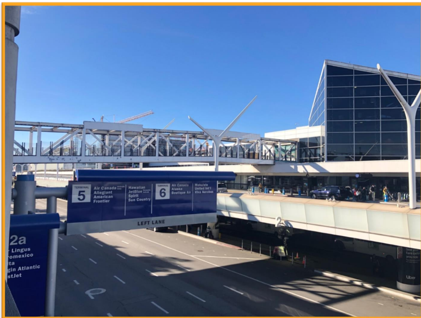
Pedestrian Bridge between Terminal 2 and Parking Structure 2A, pictured from Parking Structure 2A
